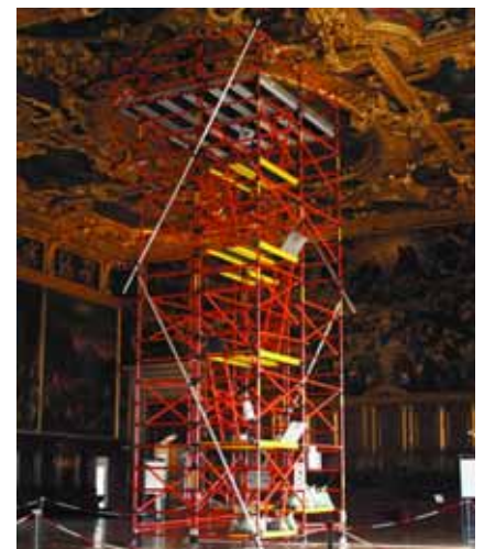
Scaffolding for the restoration work.
